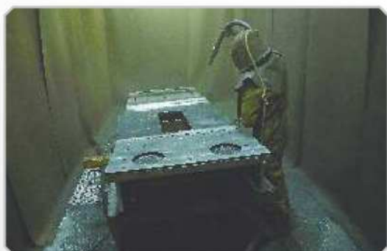
SHOT BLASTING UNIT
